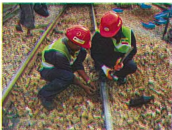
Rail Joint Work
