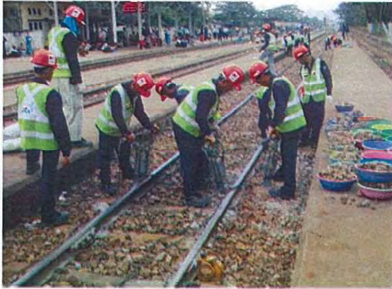
Ballast compacting work (Tie Tamper)
