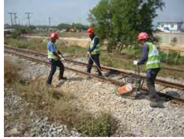
Ballast compacting work (Rammer)
