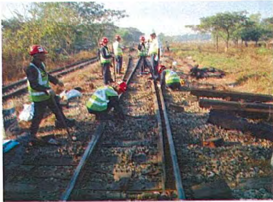
Maintenance of turnout①
