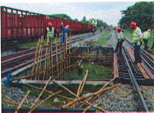
Track Maintenance on the Bridge
