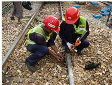
Rail Joint Work
