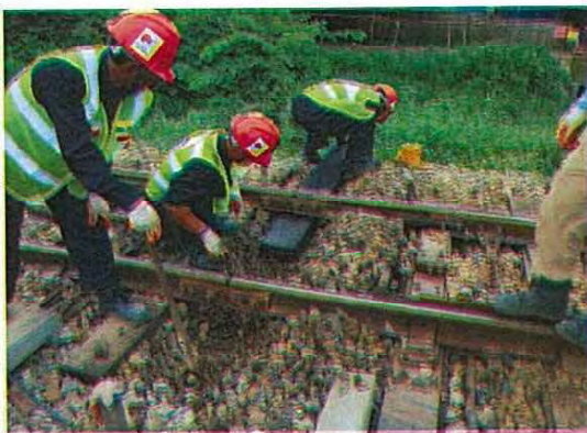
Strengthen rail joint
