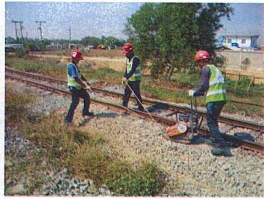
Ballast compacting work (Rammer)
