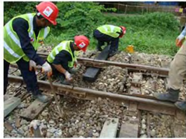
Strengthen rail joint
