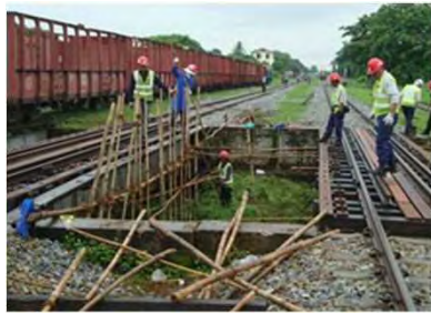
Track Maintenance on the Bridge
