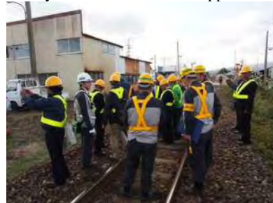
Facilities Survey under Track Possession
