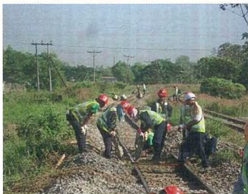
Hand Tamping at curve section
