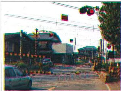
Photo 40.12 Example of overhead crossing signal
