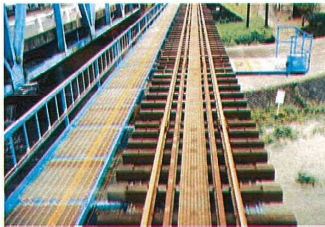
Photo 2.6.1 Example of foot plate and foot path
