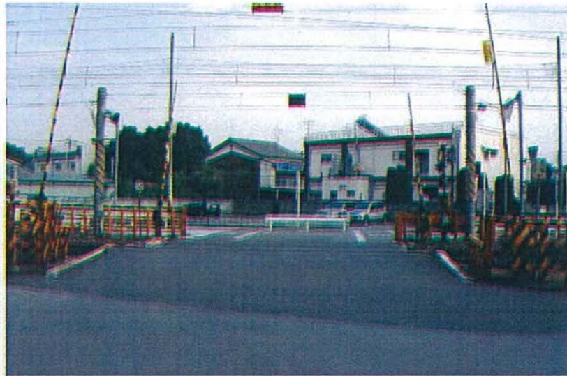
Photo 40.4 Example of asphalt paved crossing
