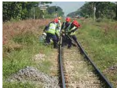
Mending alignment at curve section
