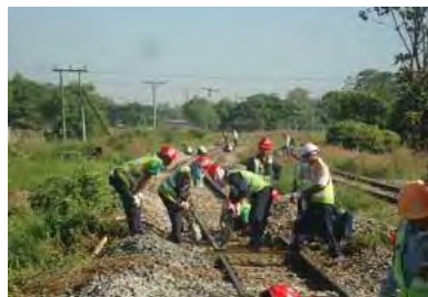
Hand Taping at curve section
