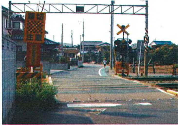
Photo 40.2 Example of Class 3 level crossing road
