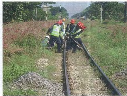
Mending alignment at curve section
