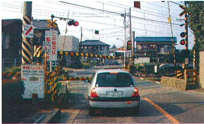
Photo 40.10 Example of double-bar barrier device
