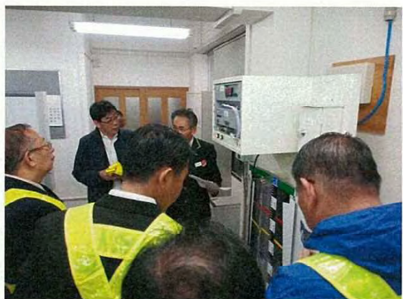
Oiwake Facilities Skill Training Center
