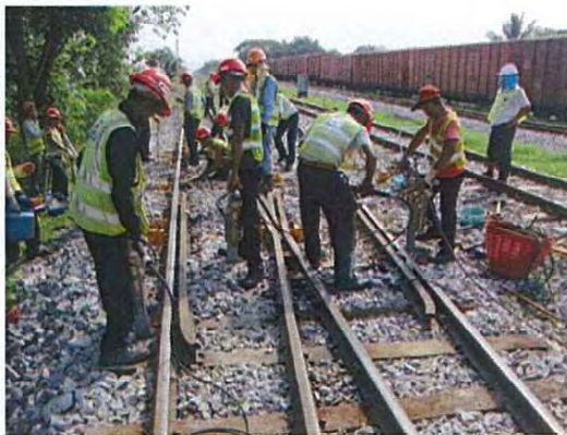
Tamping at turnout
