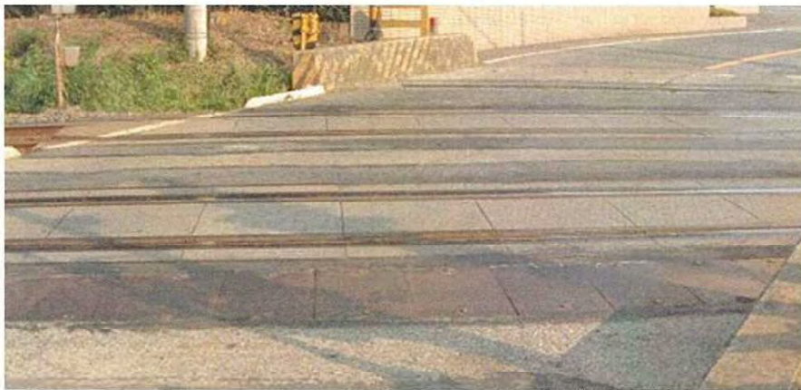
Photo 40.5 Example of concrete paved crossing
