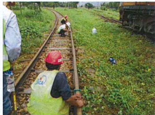
Measuring at curve section
