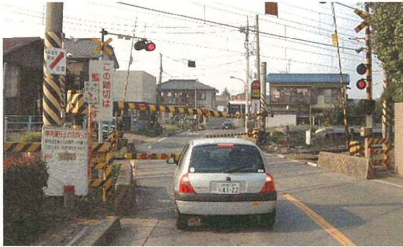
Photo 40.10 Example of double-bar barrier device
