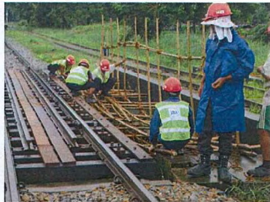
Set up scaffolding at bridge
