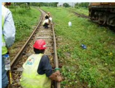
Measuring at curve section
