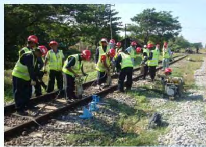
Track maintenance used by Hand Tie Tamper
