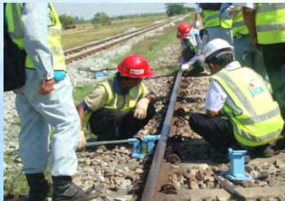
Track maintenance used by jack
