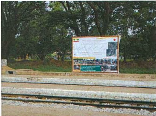
Sign Board in Toekyaungkalay Sta.
