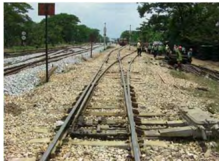
After track maintenance
