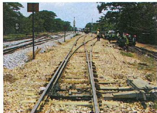
After track maintenance
