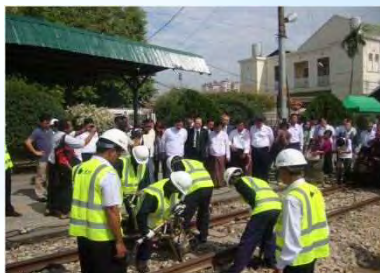
Demonstration of Hand Tie Tampers in Yangon Sta.
