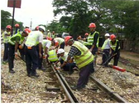
Track Raising of turnout
