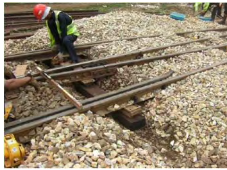
Exchanging sleeper of turnout
