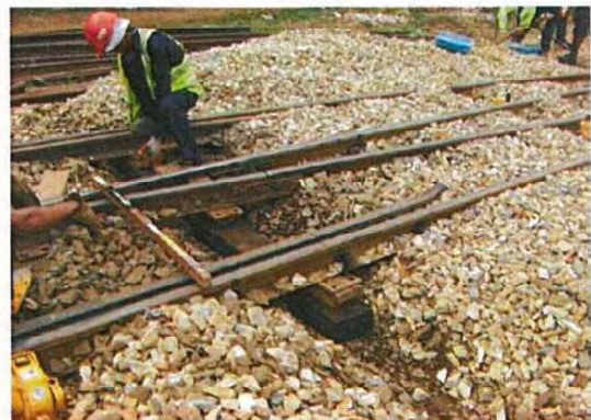
Exchanging sleeper of turnout
