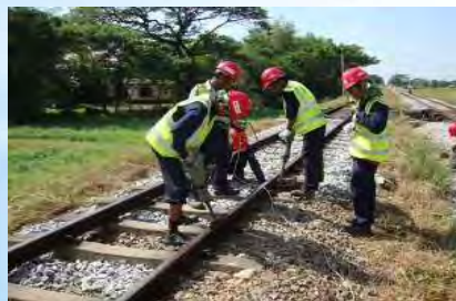
Tamping using by Hand Tie tamper of MR
