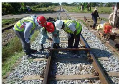
Track maintenance used by standard gauge
