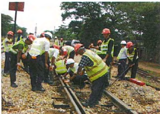
Track Raising of turnout
