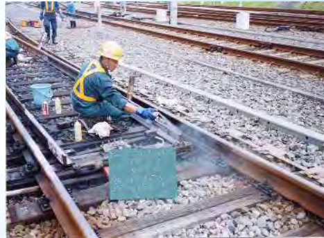
Inspection of turnout
