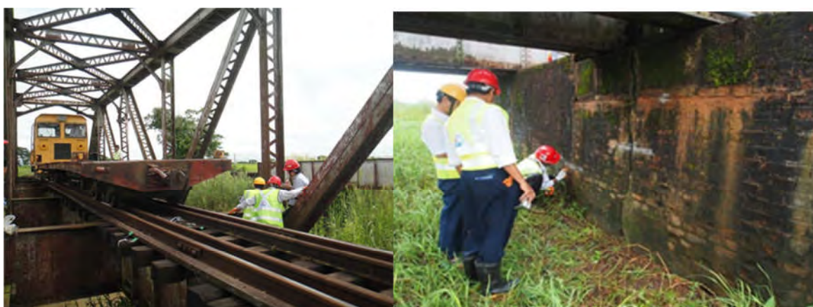
(1) Stress measure training (No32 Bridge)
