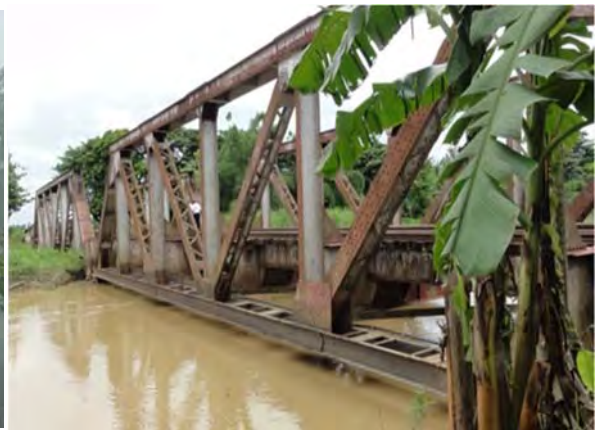
(4) Bridge (rainy season)
