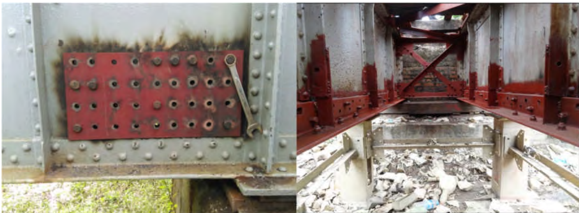
Photo 4-3 Phase2 Repairing by MR trainee
