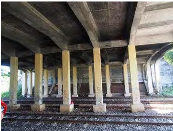
(3) Rail over bridge
