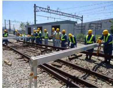
Exchange rail work in Tokyo
