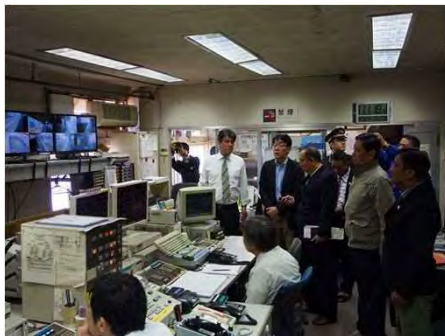
Operation Center in Akita
