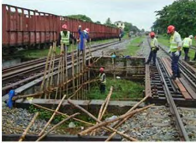
Track Maintenance on the Bridge
