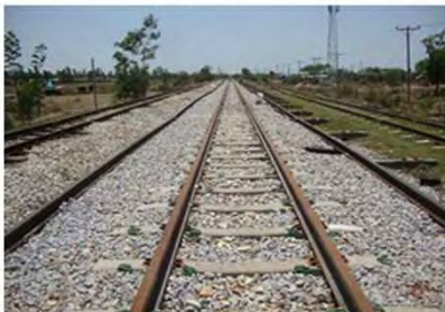
After changing 50N Rail
