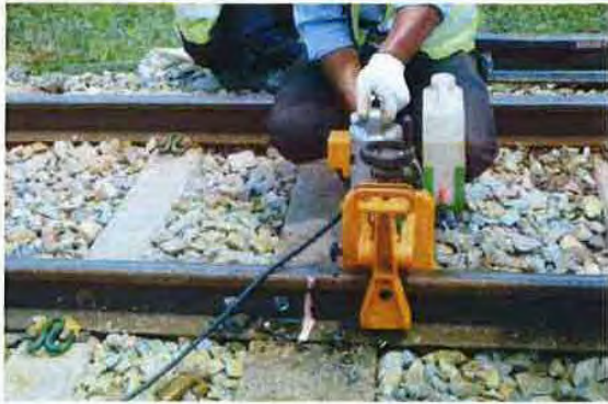
Drilling a hole of the rail
