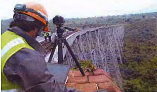
Displacement measurement on Gokteik Viaduct
