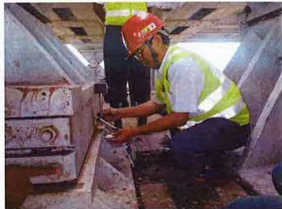
Inspection training on Inwa Bridge
