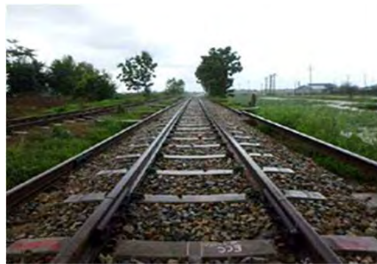
After replacing from 75lb rail to 50N rail
