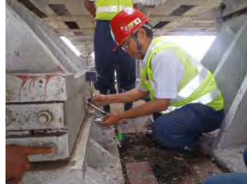
Inspection training on Inwa Bridge
