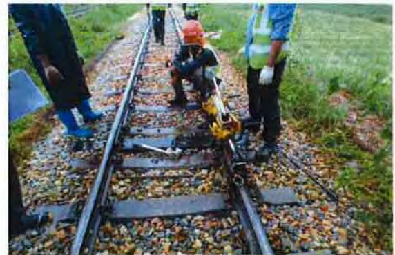
Adjustment of joint gaps
