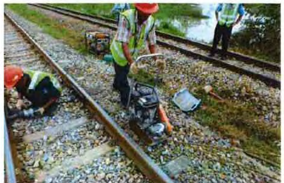
Tamping with rammer
