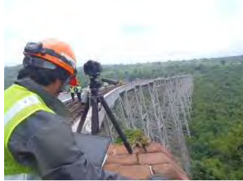
Measurement of displacement on Gokteik Viaduct
