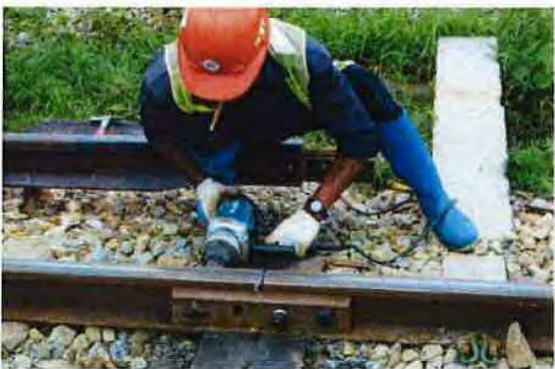
Tightening fishplates by bolts
