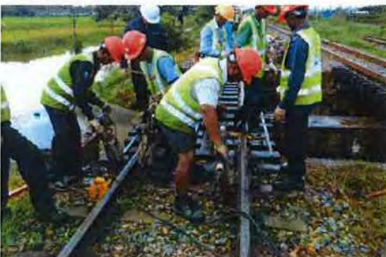
Tamping by hand tie tamper (Around bridge)
