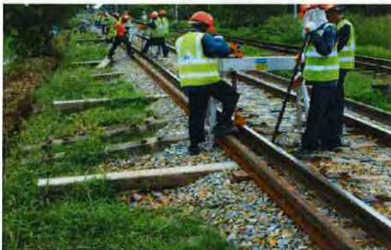
Removing 75lb Rail
