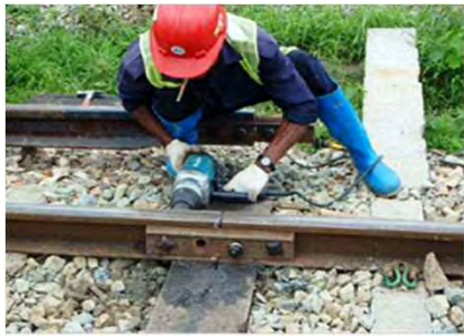
Tightening fishplates by bolts
