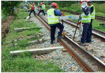
Removing 75lb Rail
