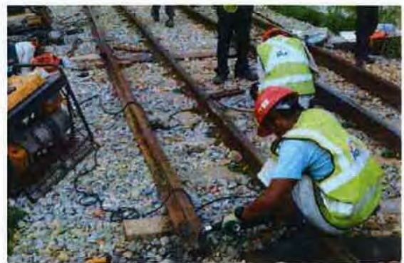
Chamfering (Removing sharp edges)
