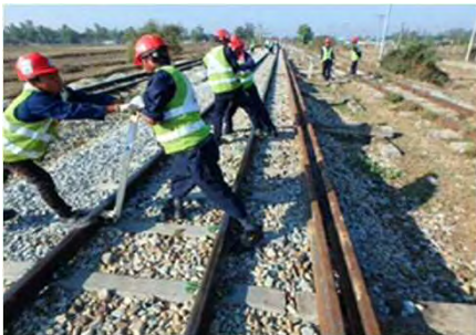
Removal of fastening (Pre-Work)
