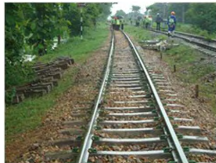
After replacing sleepers
