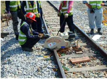
Cutting rail on the trunk line (Pre-Work)
