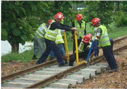
Installing fastening (First Clip)
