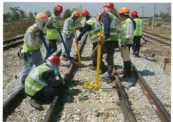
Installing fastening (First Clip)
