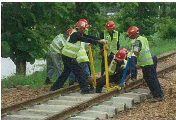
Installing fastening (First Clip)
