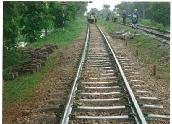
After replacing sleepers
