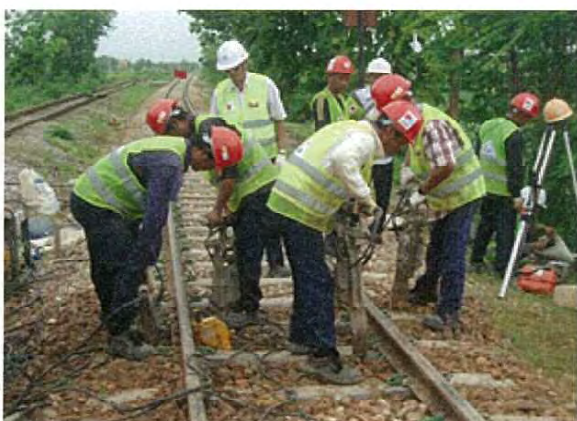
Tamping by hand tie tamper
