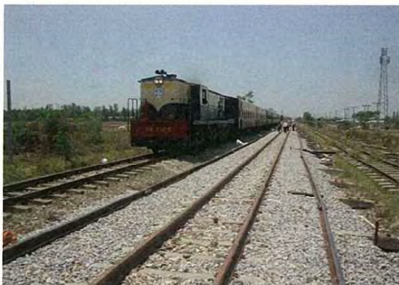
Reverse direction operation under track
