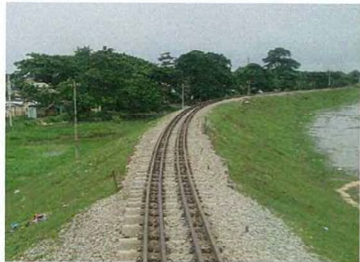
Embankment near Aungthuhka Sta.(2015)
