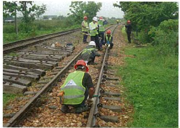
Chord-to-rail measurement
