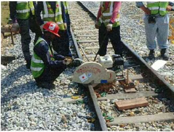
Cutting rail on the trunk line (Pre-Work)
