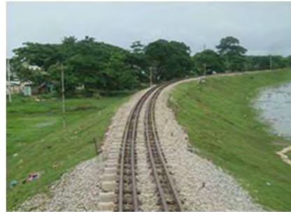
Embankment near Aungthuhka Sta.(2015)
