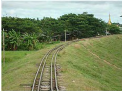
Embankment near Aungthuhka Sta.(2012)
