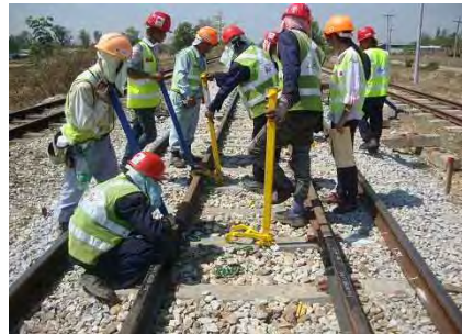
Installing fastening (First Clip)
