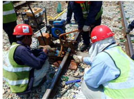
Drilling rail on the trunk line (Pre-Work)
