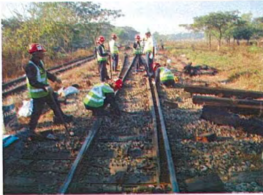
Maintenance of turnout①
