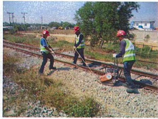
Ballast compacting work (Rammer)
