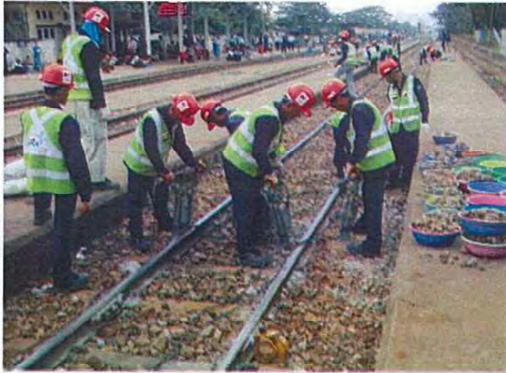
Ballast compacting work (Tie Tamper)
