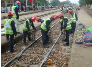
Ballast compacting work (Hand Tie Tamper)
