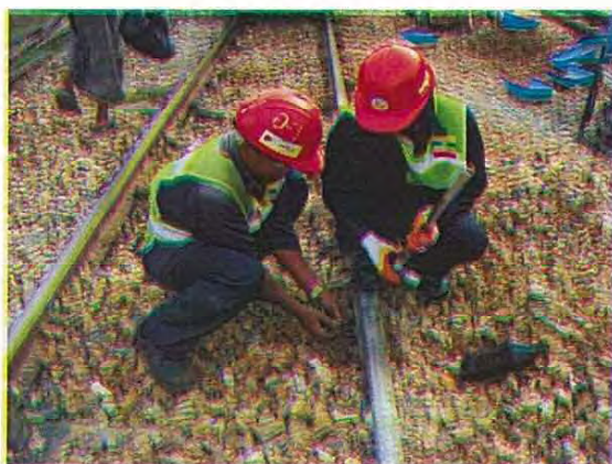
Rail Joint Work
