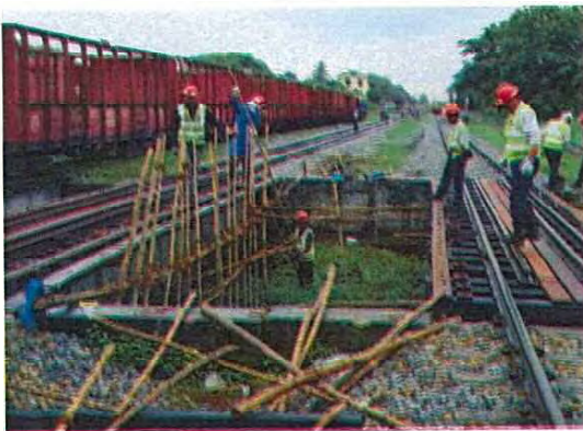
Track Maintenance on the Bridge
