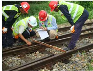
Correction of track gauge
