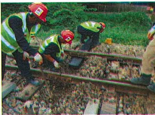
Strengthen rail joint
