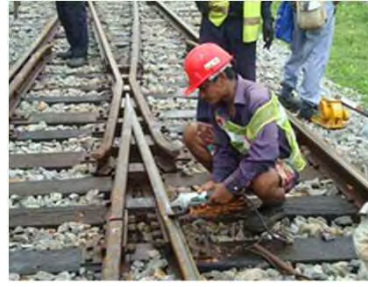
Maintenance of turnout②
