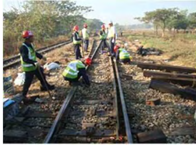
Maintenance of turnout①
