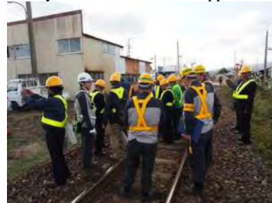
Facilities Survey under Track Possession
