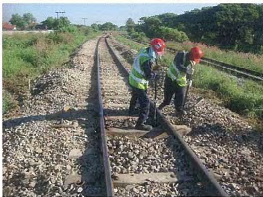
Adjustment of sleeper
