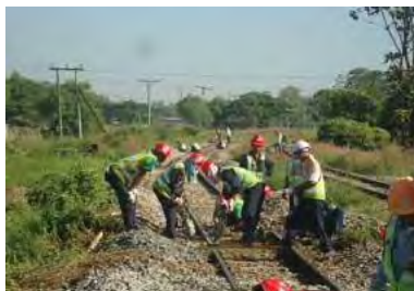
Hand Taping at curve section
