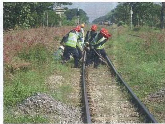
Mending alignment at curve section
