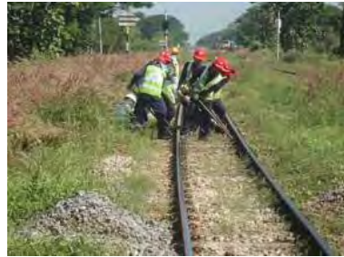
Mending alignment at curve section
