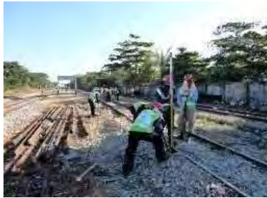
Inside station yard
