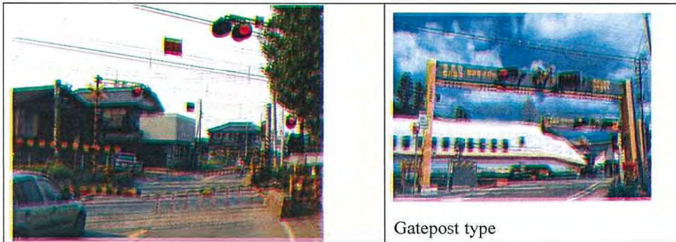
Photo 40.12 Example of overhead crossing signal
