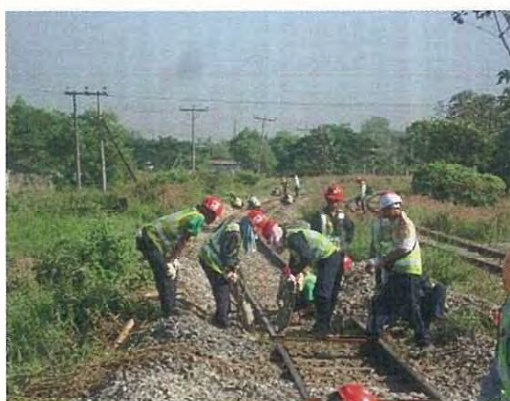
Hand Tamping at curve section
