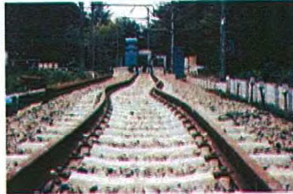
Photo 2.1.11. Long welded rail buckling test at JR Technical Research Institute
