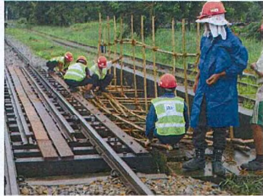
Set up scaffolding at bridge
