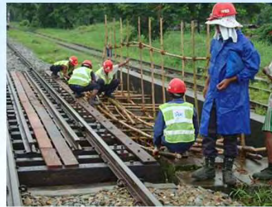
Set up scaffolding at bridge
