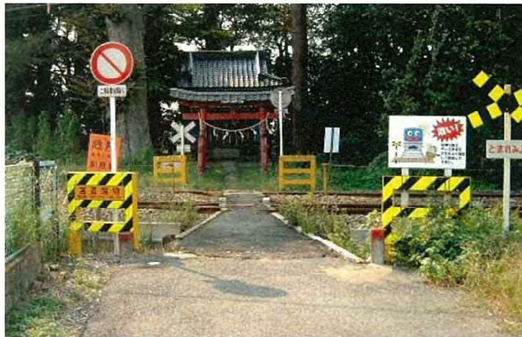
Photo 40.3 Example of Class 4 level crossing road
