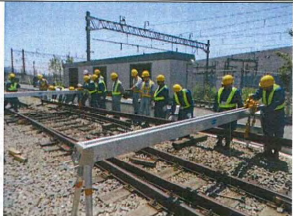
Replacement of Rail
