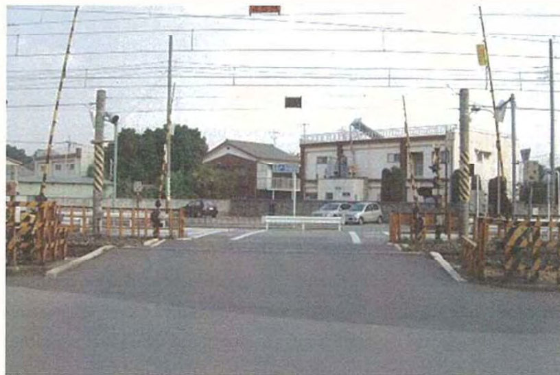
Photo 40.4 Example of asphalt paved crossing
