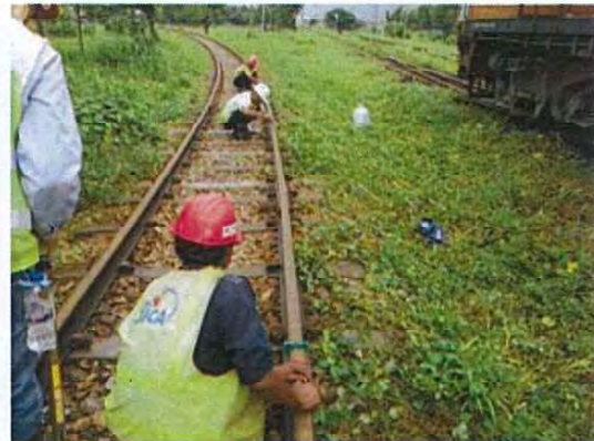
Measuring at curve section
