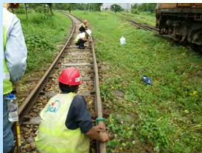
Measuring at curve section
