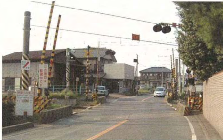
Photo 40.1 Example of Class 1 level crossing road
