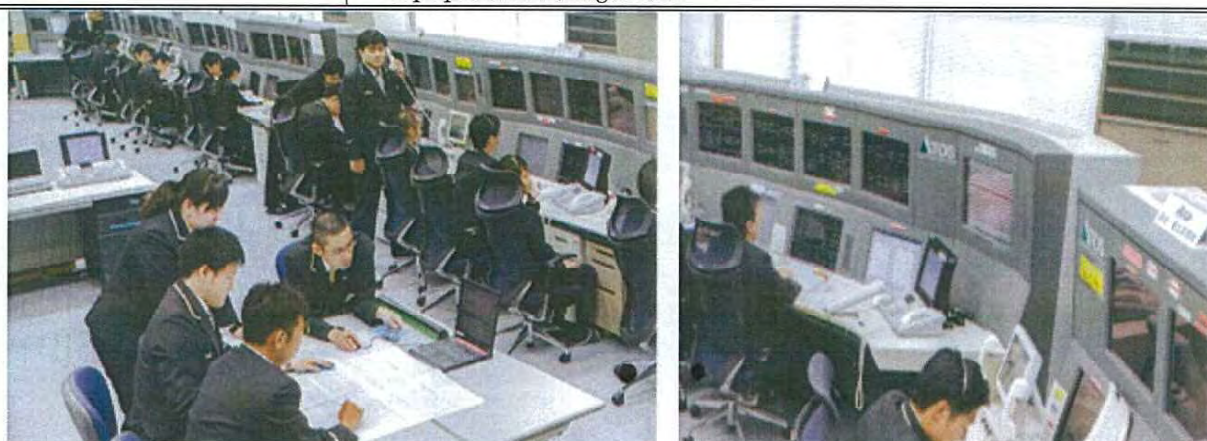
Tokyo Operation Control Center
