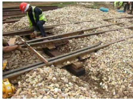
Exchanging sleeper of turnout
