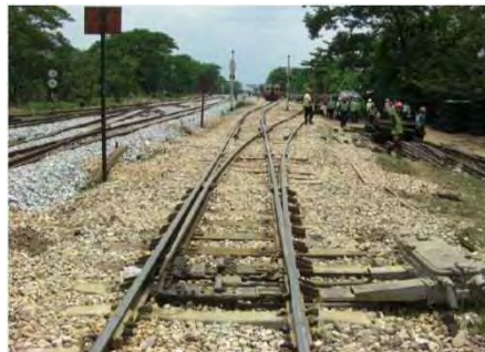
After track maintenance
