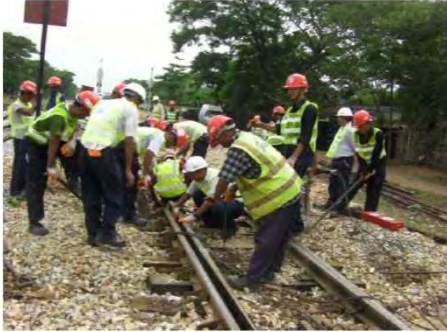
Track Raising of turnout
