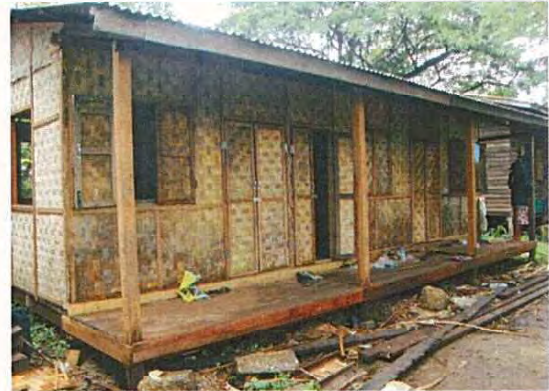
Temporary Dormitory for trainee
