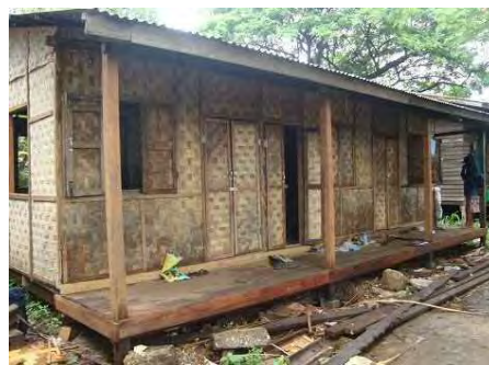
Temporary Dormitory for trainee
