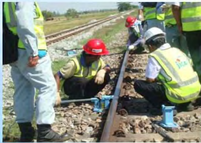
Track maintenance used by jack
