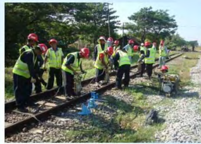
Track maintenance used by Hand Tie Tamper
