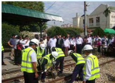
Demonstration of Hand Tie Tamper in Yangon Sta.
