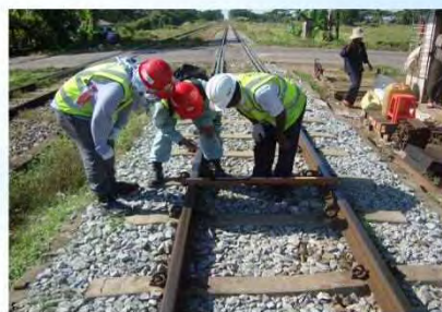
Track maintenance used by standard gauge
