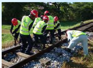
Track maintenance by man power
