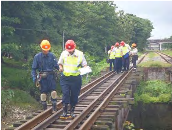
(1) No9 Bridge 検査の着眼点訓練
