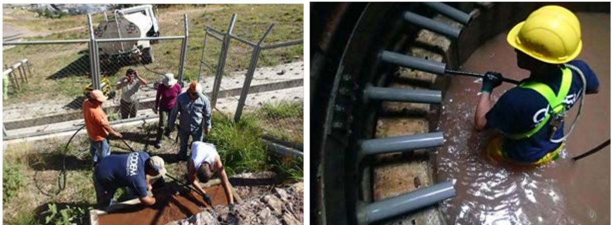
Figure 11 Clearing the clogged pipes of horizontal drainage (Source: JCT)
