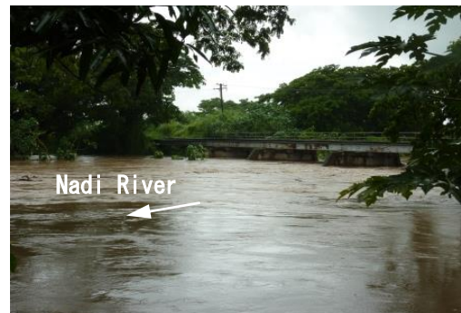
Photo-12 Nadi River (Old Queens Road Bridge) during Flood
