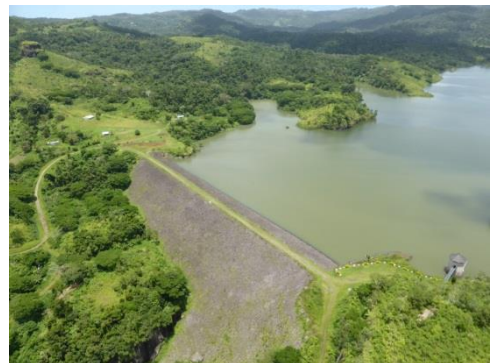
Photo-8 Vaturu Dam (Nadi River Upstream)
