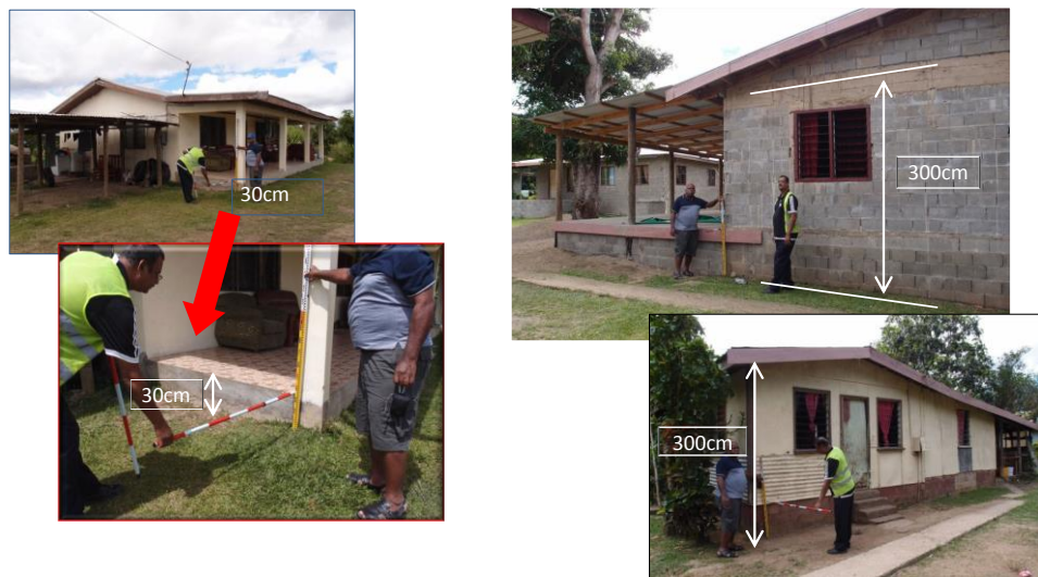
Figure 7-31 Field Survey of Housing in Objective Area
