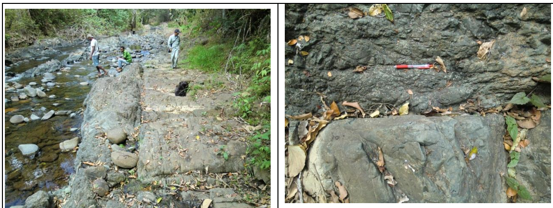
Photo 6-14 Condition of Geology and Bed Rock (River bed of NAW-1)
