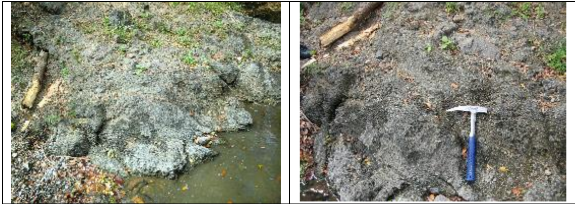
Photo 6-4 Condition of Geology and Bed Rock (River bed of NAD-2 )
