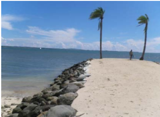
Picture8-1 Left Side of Jetty at NAISOSO
