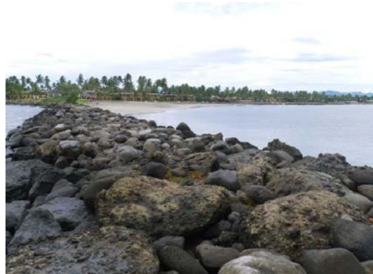
Picture2-2 Stone Jetty at Denarau Sheraton
