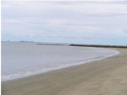
Picture2-1 Stone Jetty at Denarau Sheraton
