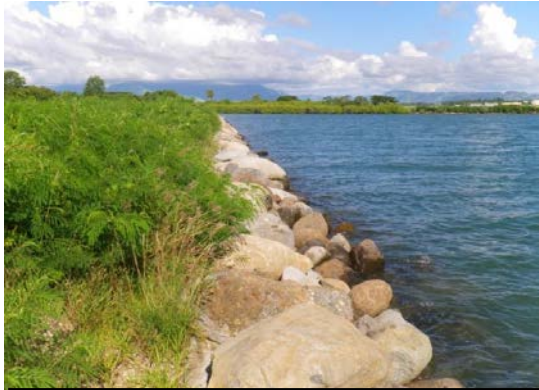
Picture7-1 Left Side of Jetty at NAISOSO
