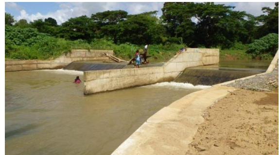
Photo-14 Retention Dam (Nawaka River)
