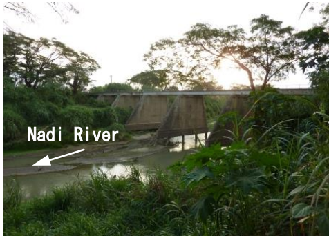
Photo-11 Nadi River (Old Queens Road Bridge)
