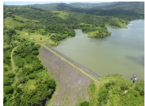
Photo-8 Vaturu Dam (Nadi River Upstream)
