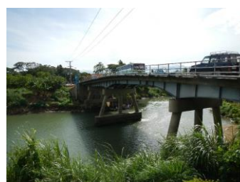
Photo 15-1 Current View (from lower left bank)
