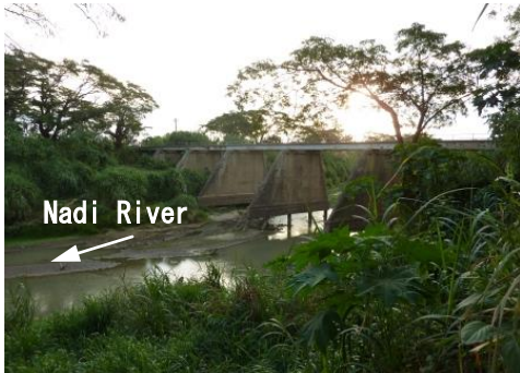
Photo-11 Nadi River (Old Queens Road Bridge)
