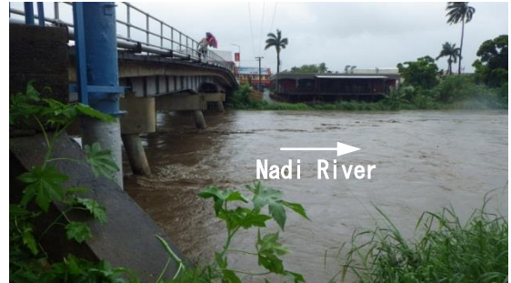
Photo-10 Nadi River (Nadi Town Bridge) during Flood
