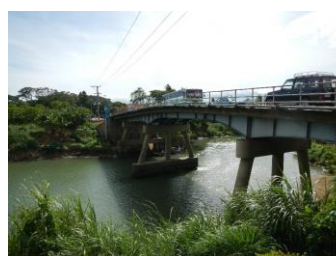
Photo 15-1 Current View (from lower left bank)
