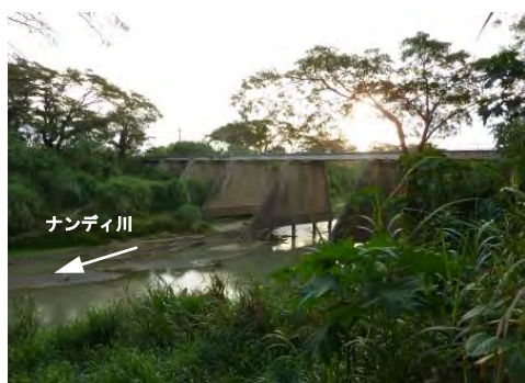
写真-11 ナンディ川 (Old Queens Road Bridge)
