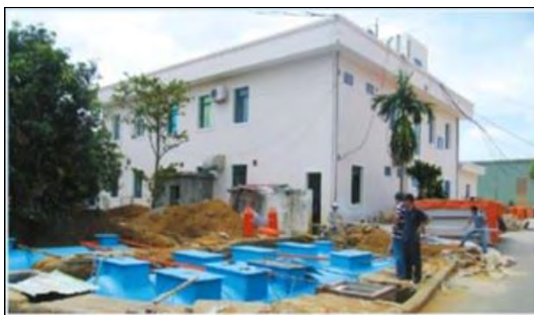
Figure 7-32 Example for Pre-Fabricated FRP Packaged On-Site Wastewater Treatment
