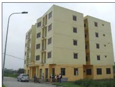
Figure 3-7 Example of the Residential Units Converted from Ex-Single Type Dormitory to Family Type (Dai An IP)
