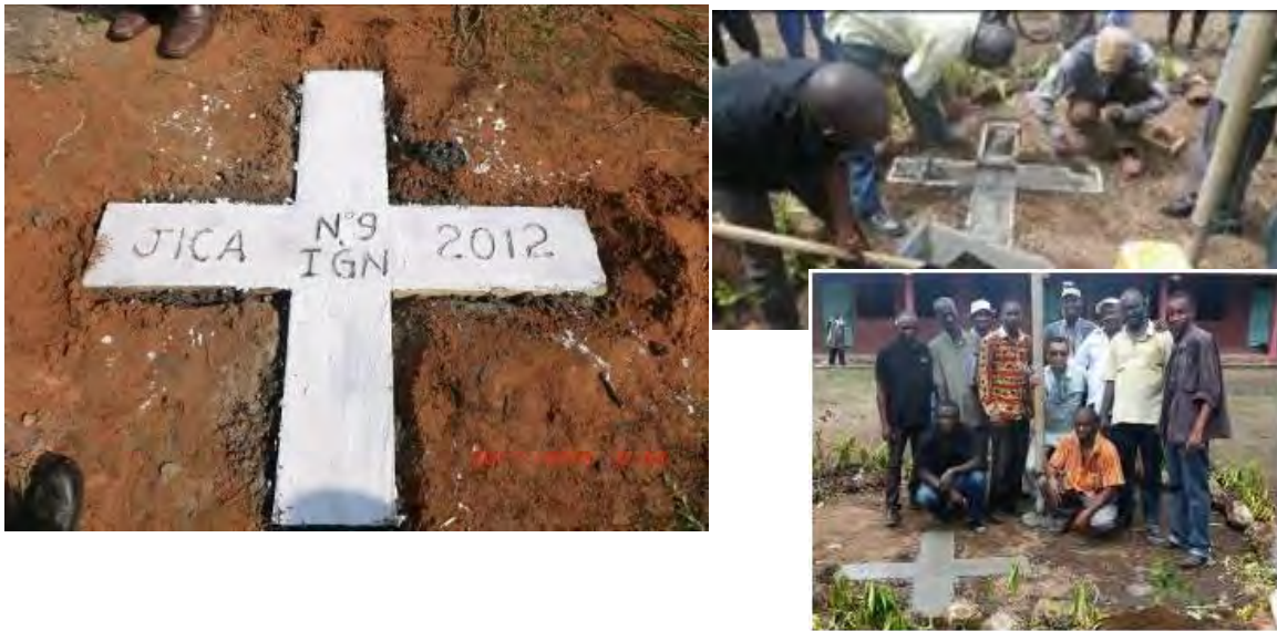
Photo 2-1 Installation of an Aerial Marker
