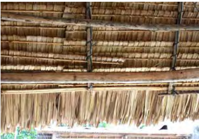
Photo 1-9: Nipa Shingles for roofing.
