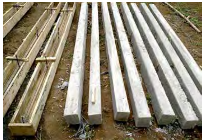
Photo 1-14: "Home-made" cement pillars
