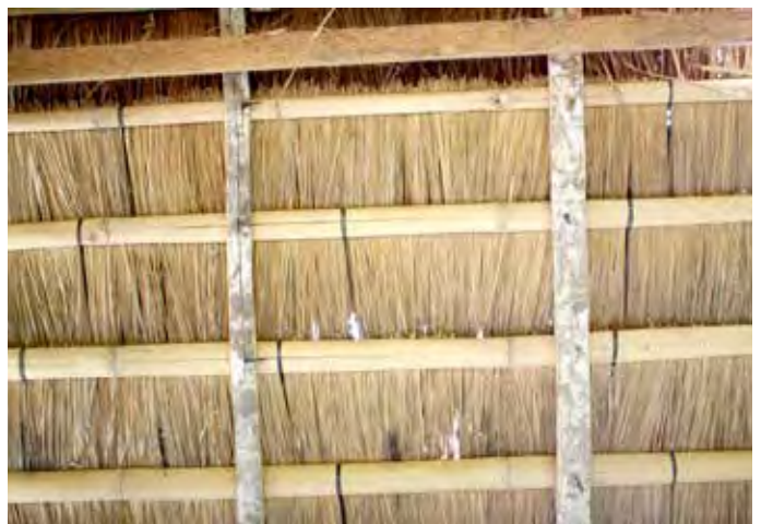
Photo 1-10: Cogon (Gie) for roofing.
