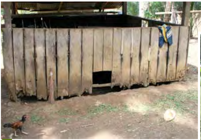
Photo 1-1: A house under the owner's house.
