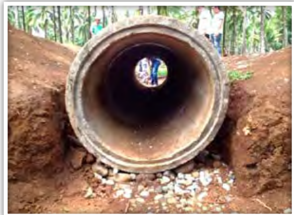
Figure 24: Culvert Bedding (cross-section in between collars)
