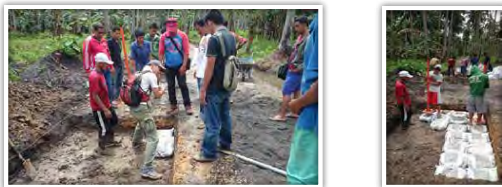
Figure 29: Do-Nou Method Actual Application
