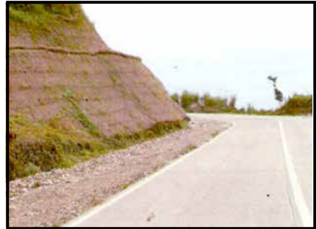
CocoNet Slope Protection
