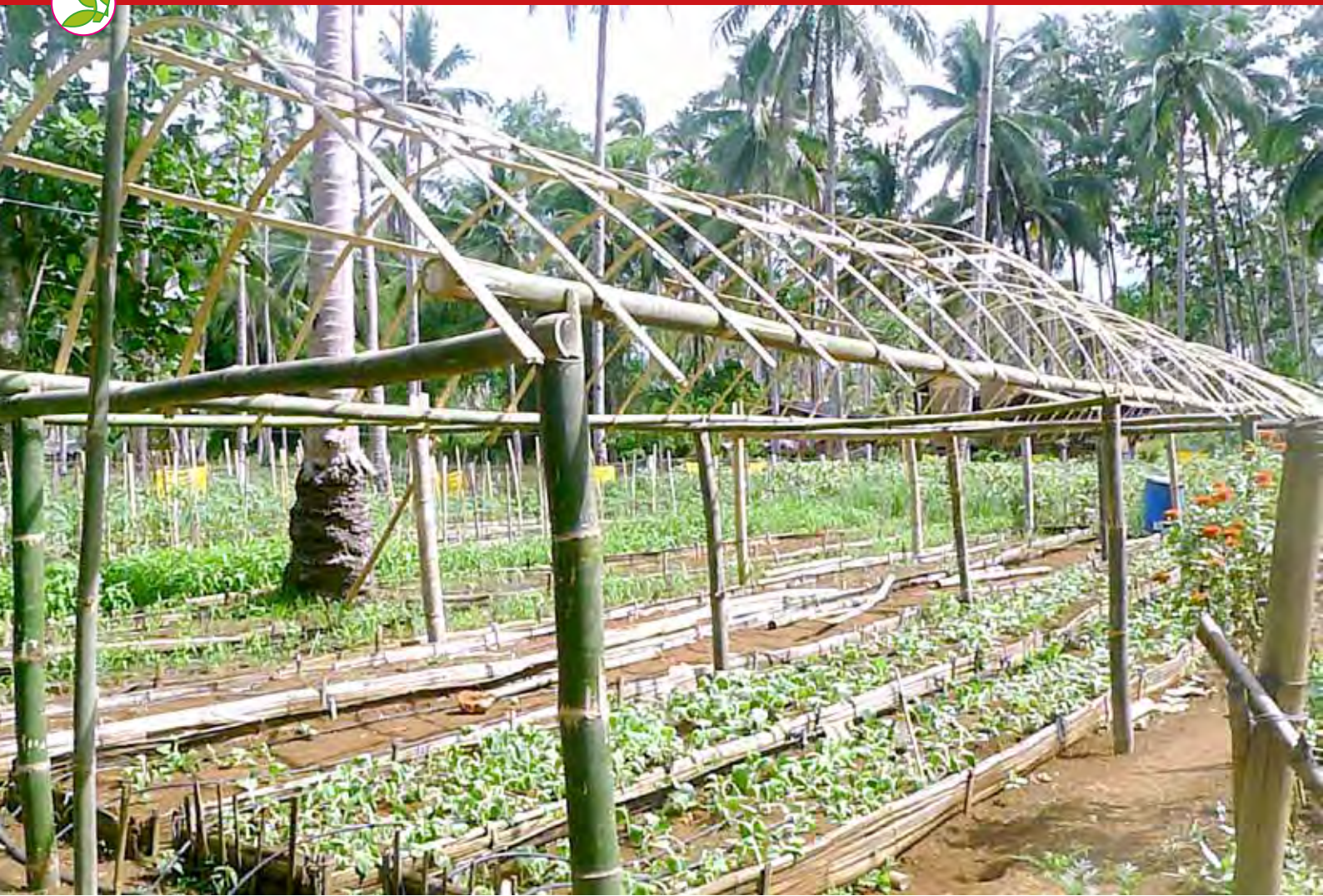
Frame of rain shelter
