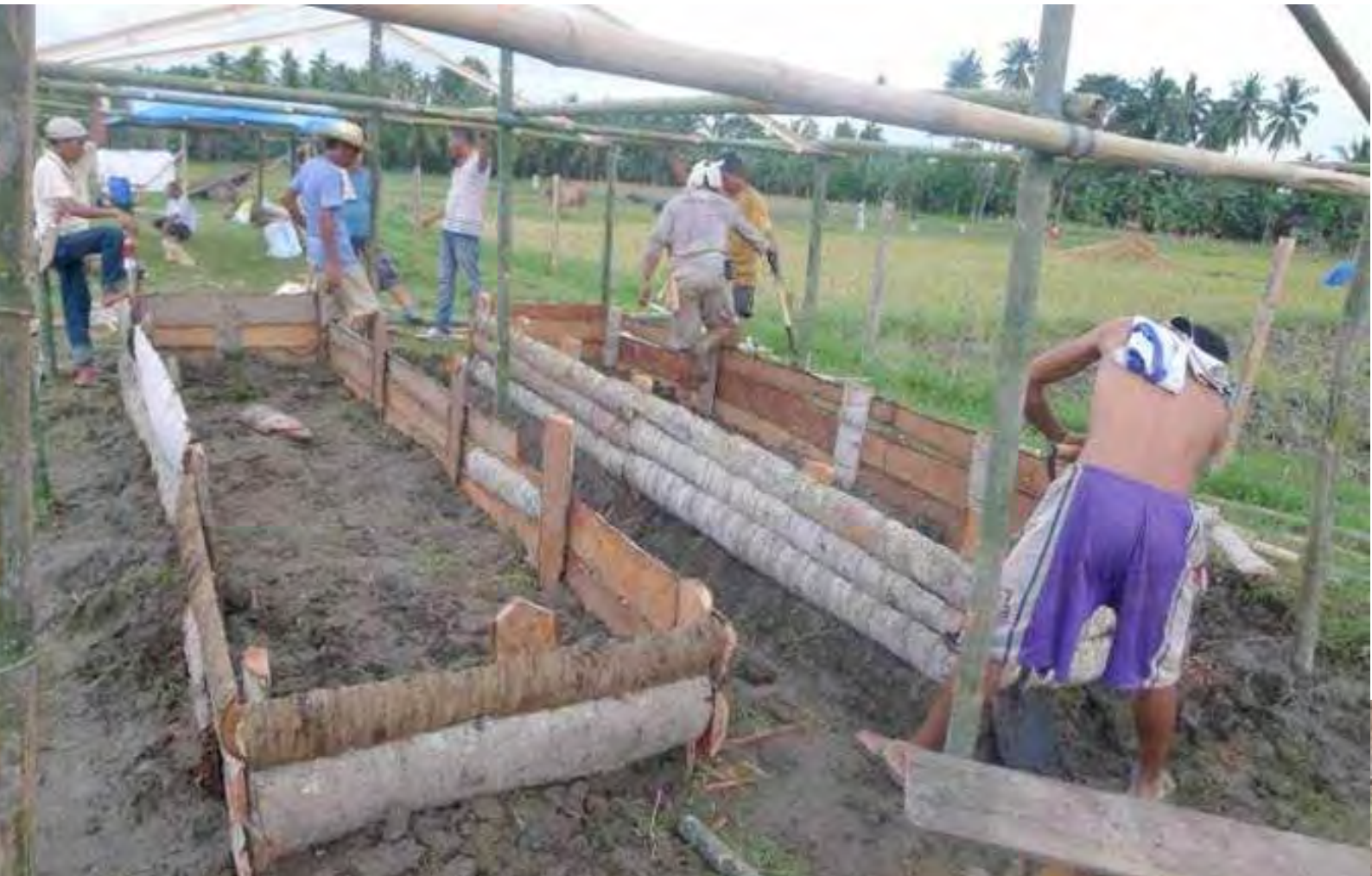
Vermi-beds construction by use of coconut trunks
