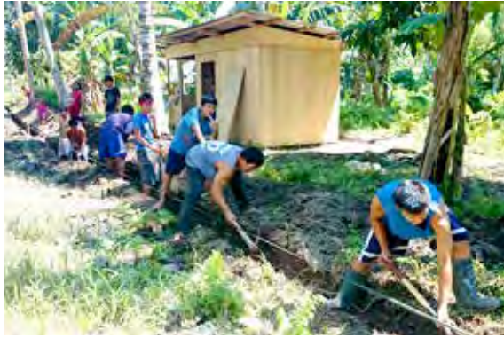
Road work by the Pakyaw group
