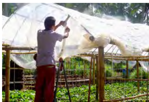
Installing a rain shelter
