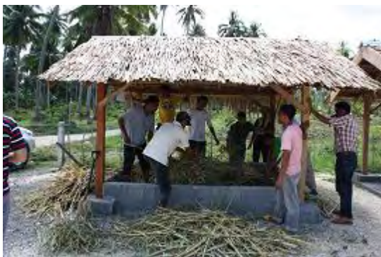
Figure 3.2.3.9: Shed for vermi-compost in Sultan Mastura
