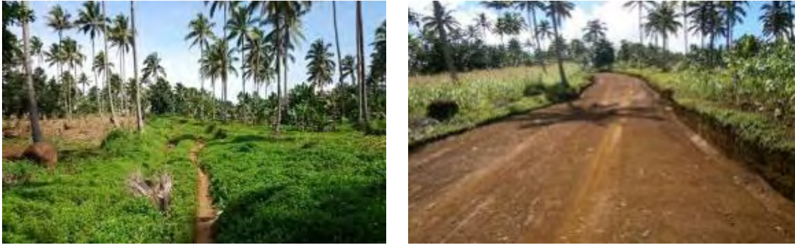
Figure 3.1.3.6: Before and after clearing
