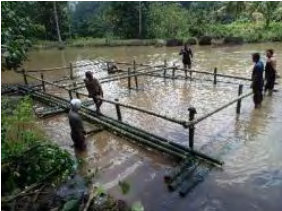
Construction of bambo floating cage (Pasayanon, March 2014)
