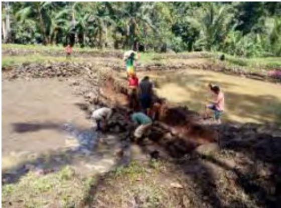
Construction and rehabilitation work of fish ponds
