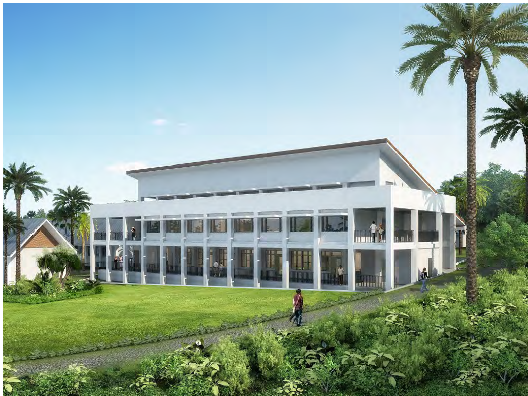
Figure III : Image of North Side
