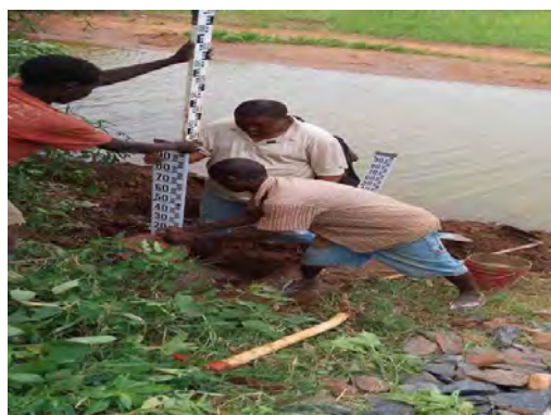
Figure P.3: Construction of the Water Level Gauges at Gulwe
