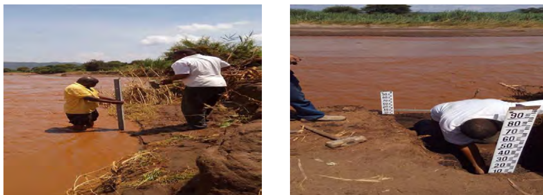
Figure P.9: Constructing the Water Level Gauges at Mbori
