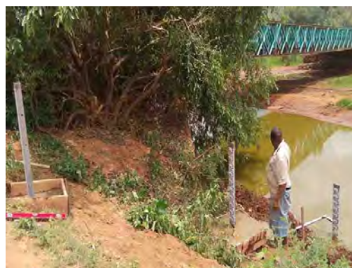
Figure P.3: Construction of the Water Level Gauges at Gulwe
