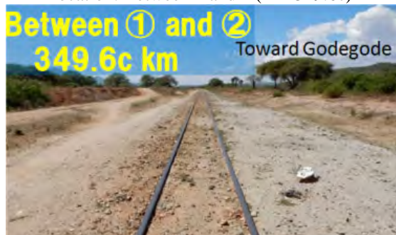
Location: Between 1 and 2 (Km 349.6c)
