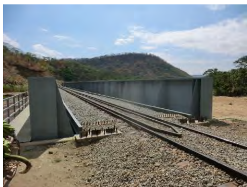
Figure 10.40: Steel Through Girder Bridge with a Maintenance Passage of 1.0 m Width on the Upstream
