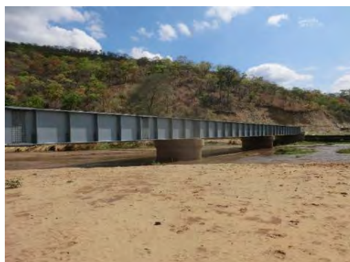
Figure 10.40: Steel Through Girder Bridge with a Maintenance Passage of 1.0 m Width on the Upstream
