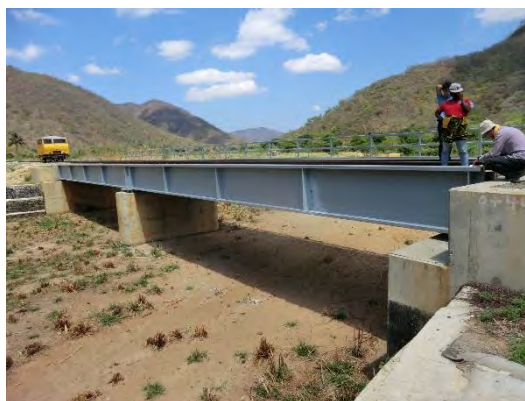
Figure 10.22: Existing Steel Deck Girder Bridge (Km 304.3)
