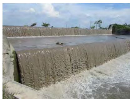
B: Mud Flow Flowing from Consolidation Dam (Indonesia)
