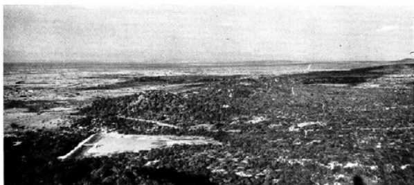
Imagi Dam Full View (December 1970)
