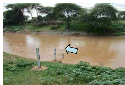
B: Water Level Gauging Station
