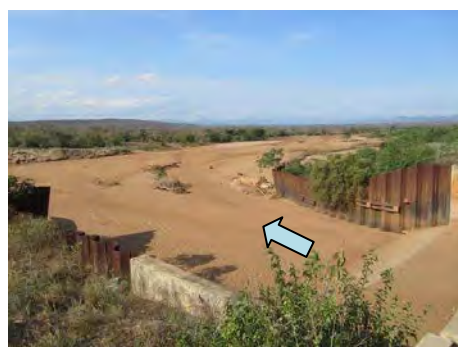
A: Existing Channel Works (Condition of Confluence)
