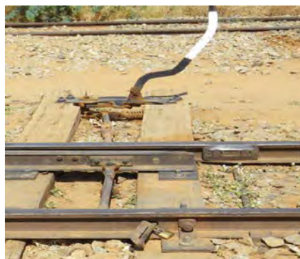
Figure 9.18: Manually-turned Point (Locked with a Padlock)
