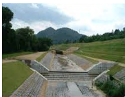
D: River Channel Works
