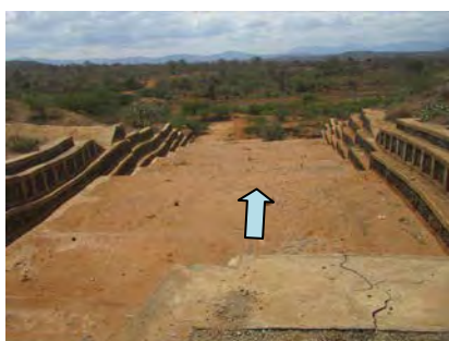
A: Channel Works at the Upstream Side
