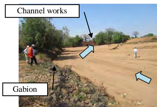
C: Revetment Works along Left Bank
