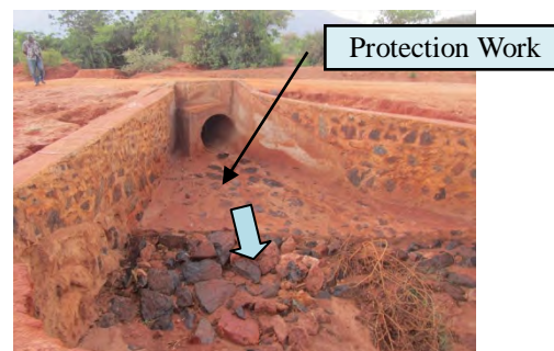
B: Road Culvert
