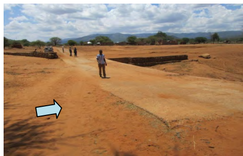
C: Road having Consolidation Dam Function
