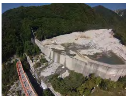
C: Check Dams
