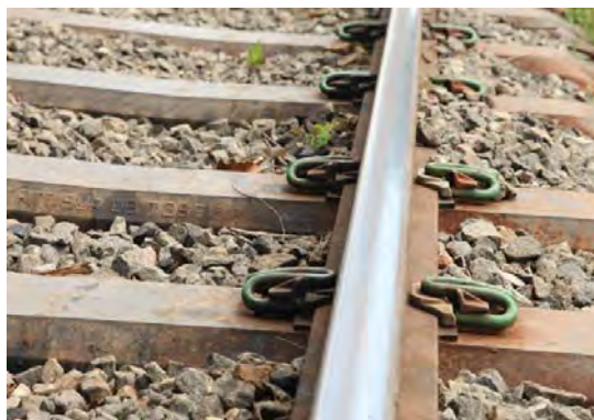
Figure 9.35: Rail Fastener
