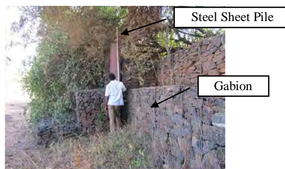
D: Revetment Works along Left Bank
