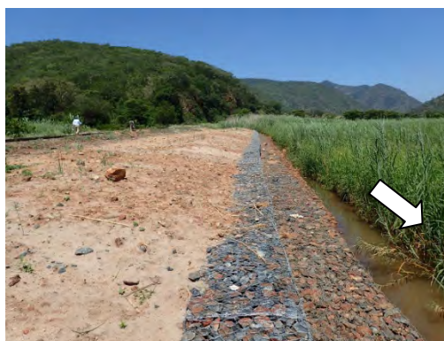
Figure 5.10: Completed Revetment by Gabion at Km 302
