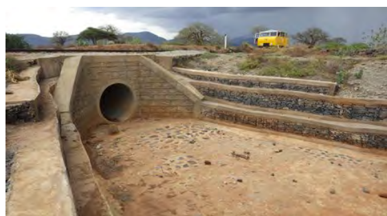
Figure 3.14: Circular Culvert (Km 349)
