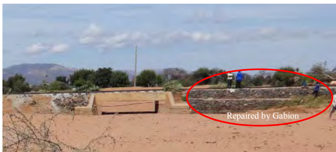
Figure 6.46: Example of Culvert Intake
