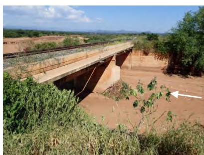
Figure 5.20: Kidibo Bridge (Railway)
