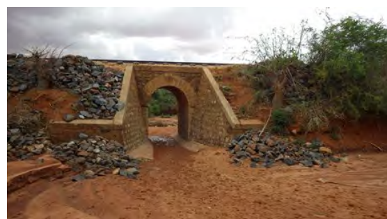
Figure 3.15: Arched Culvert (Km 410)
