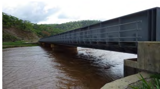
Figure 3.12: Steel through Bridge (Km 293)
