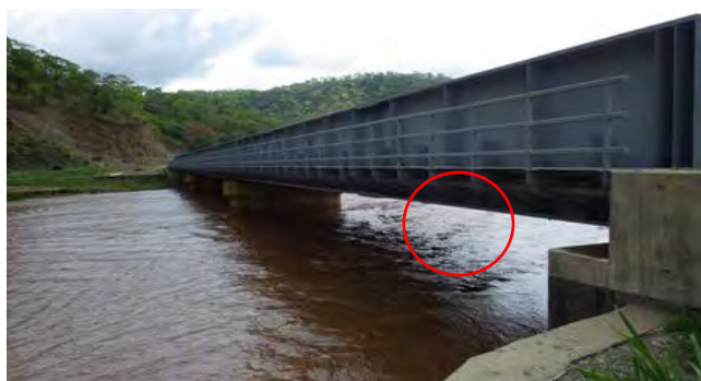
Figure 3.17: Danger Point of the Bridge Destruction (Km 293)
