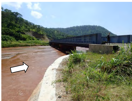
Figure 5.9: Completed New Bridge at km 293
