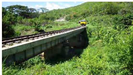
Figure 3.11: Steel Girder Bridge (Km 292)
