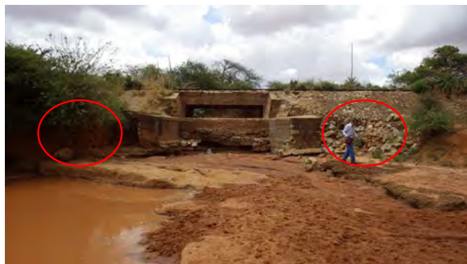
Figure 3.16: Embankment Erosion by Running Water (Km 410)
