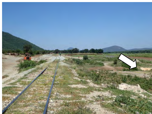
Figure 5.11: Completed Shifting of Railway Alignment at Km 315
