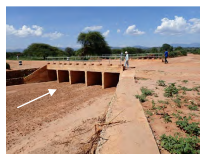
Figure 5.18: New Box Culvert Constructed by TANROADS
