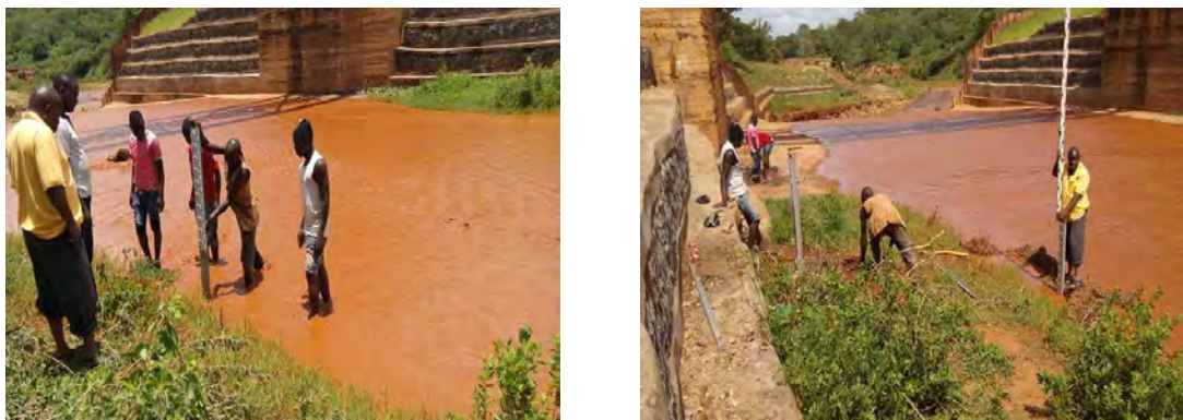
Figure P.7: Construction of the Water Level Gauges at Kidete
