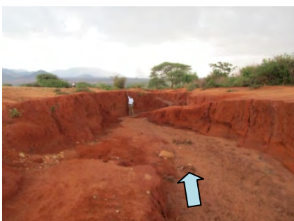
A: Eroded Road Gutter
