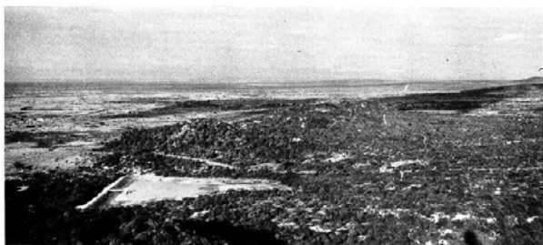
Imagi Dam Full View (December 1970)
