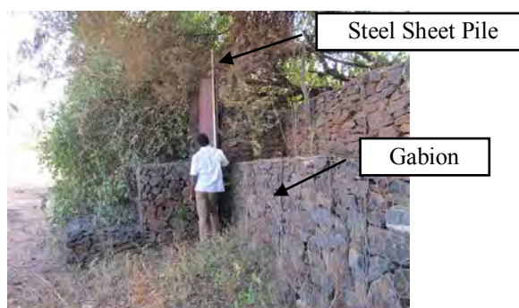
D: Revetment Works along Left Bank
