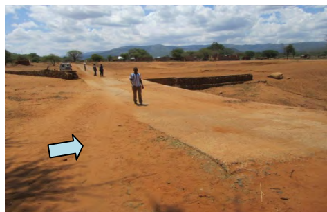
C: Road having Consolidation Dam Function
