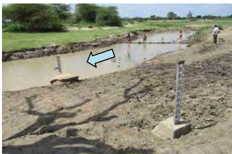
A: A Small Amount of Sediment Deposition
