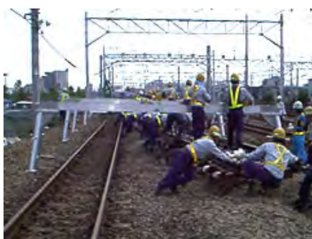
Figure 9.31: Special Over-Raise Rail Shifter for Heavy Articles
