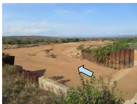
A: Existing Channel Works (Condition of Confluence)
