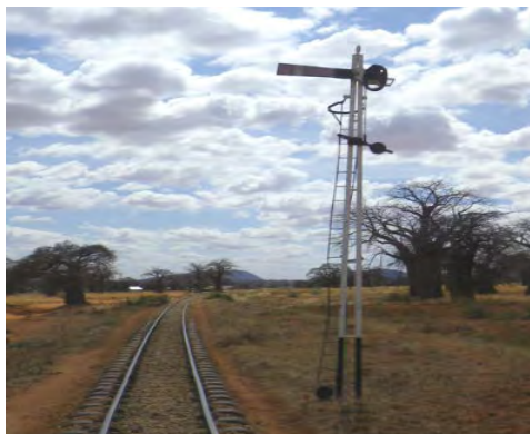
Figure 9.17: Semaphore Signals (Destroyed and Not in Use)
