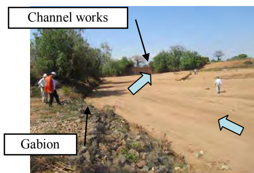
C: Revetment Works along Left Bank
