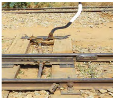
Figure 9.18: Manually-turned Point (Locked with a Padlock)
