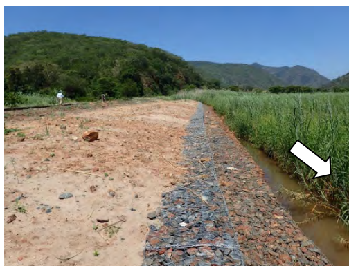
Figure 5.10: Completed Revetment by Gabion at Km 302
