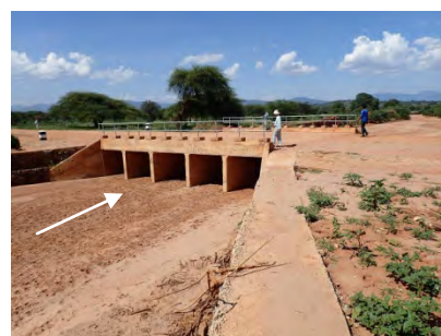
Figure 5.18: New Box Culvert Constructed by TANROADS
