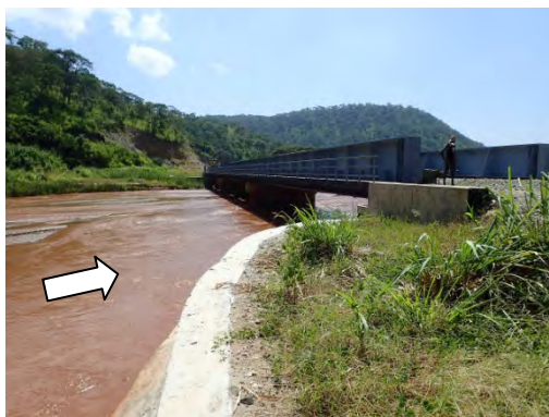
Figure 5.9: Completed New Bridge at km 293
