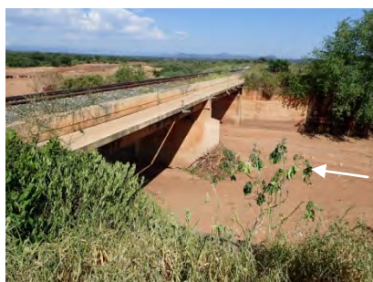
Figure 5.20: Kidibo Bridge (Railway)
