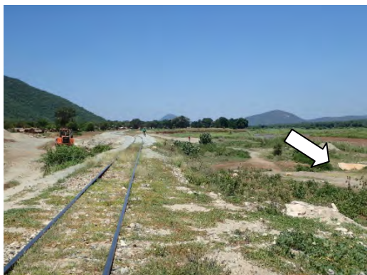
Figure 5.11: Completed Shifting of Railway Alignment at Km 315
