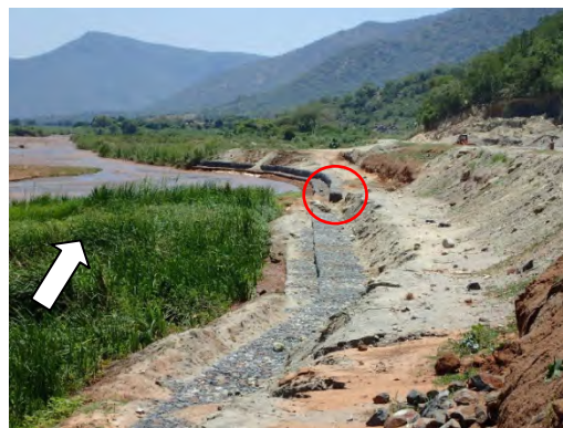
Figure 5.12: Suspension of Installation Works of Gabion
