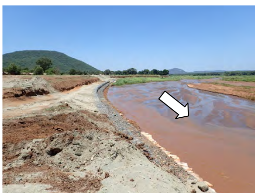
Figure 5.13: Completed Feature of Revetment Works by Gabion Boxes (Lower Level)
