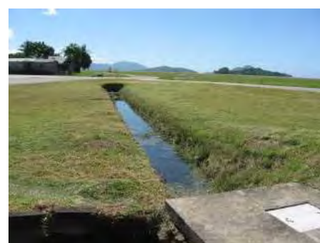
Photo 5-2-16: Airport drainage channel (C) (April 2011)
