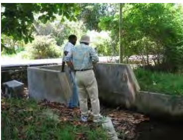
Photo 5-2-26: Inlet of Pipes (April 2011)
