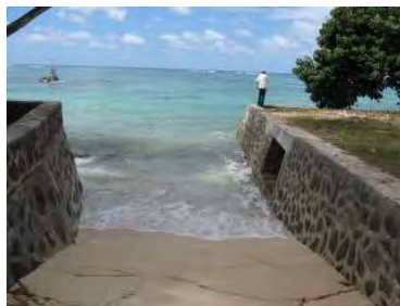
Photo 5-2-23: Outlet D is not in Water (May 2011)
