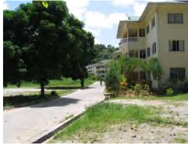
Photo 5-2-20: Residential Development at Remy Estate (April 2011)
