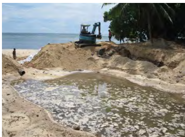
Photo 5-2-27: Outlet C, under improvement (Jan 2014)
