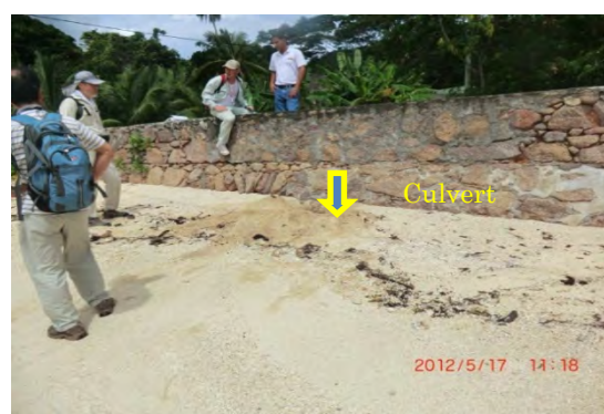
Figure 6-6-16: Drainage by Three Pipes (2012) Figure 6-6-17: Clogging of Culvert (17/5/2012)
