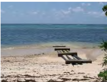
Photo 5-2-25: Outlet C Discharge by Pipes (April 2011)
