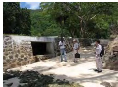
Photo 5-2-24: Outlet D (April 2011)
