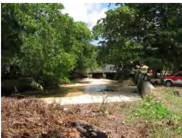
Photo 5-2-22: Outlet B Reduced width of Outlet (April 2011)
