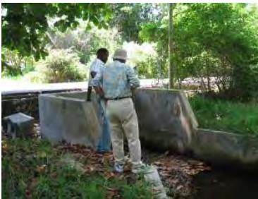
Photo 5-2-17: Inlet of Pipes (April 2011)
