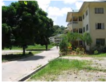
Photo 5-2-11: Residential Development at Remy Estate (April 2011)
