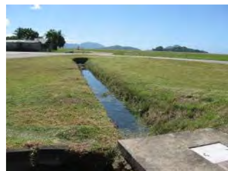
Photo 5-2-7: Airport drain channel (C) (April 2011)
