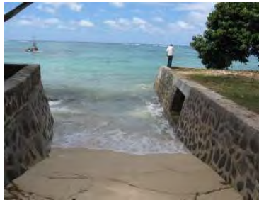
Photo 5-2-14: Outlet D is not in Water (May 2011)
