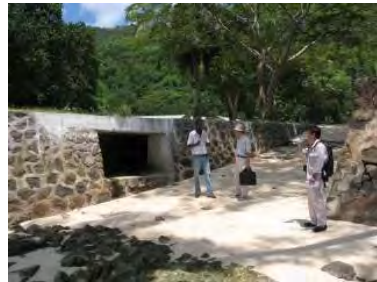
Photo 5-2-15: Outlet D (April 2011)
