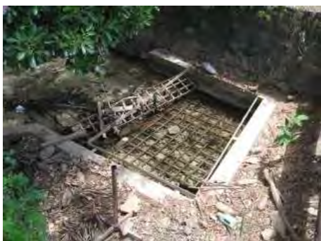
Photo 5-2-8: Outlet of Wetland (May 2011)
