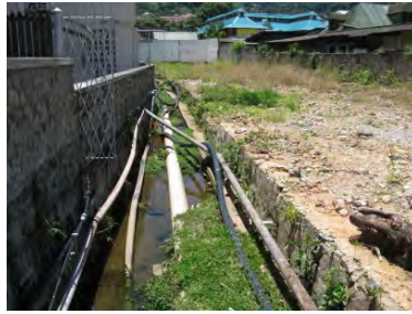
Photo 5-2-2: Obstacle in River Maintry
