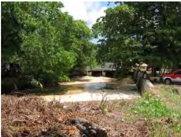
Photo 5-2-13: Outlet B Reduced width of Outlet (April 2011)
