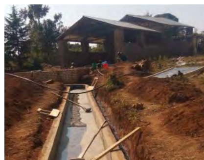
CPU building and facilities
