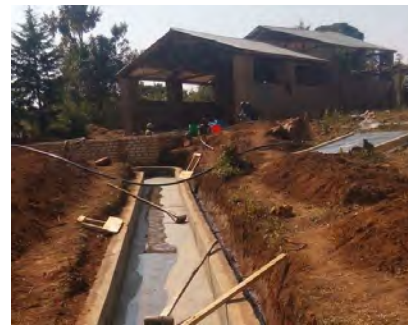
CPU facility completed with loan
