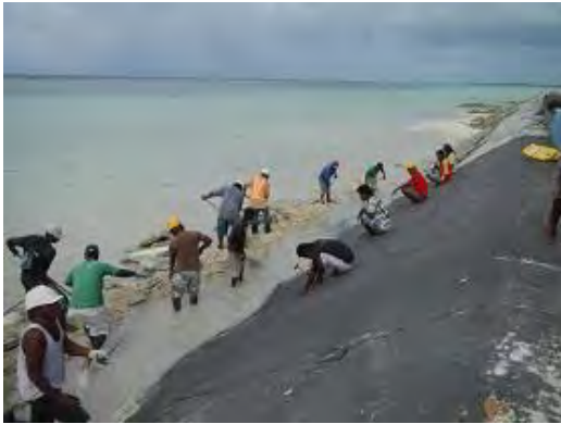
Installation of geotextile sheets
