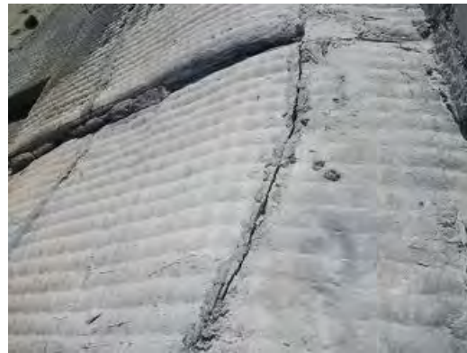
Peeling after application of mortar due to poor workmanship
