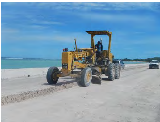
Scraping and filling by motor grader
