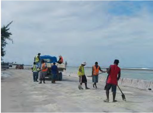
Filling while walking with a dump truck
