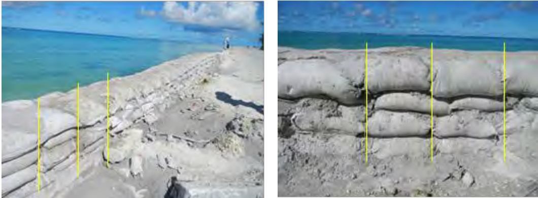
Sandbags are piled in one column (not alternately piled)
