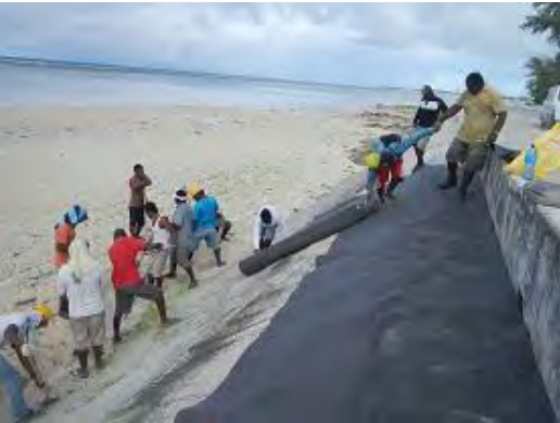
Installation of geotextile sheets
