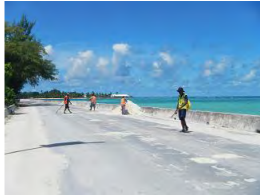
Filling pot holes by workers
