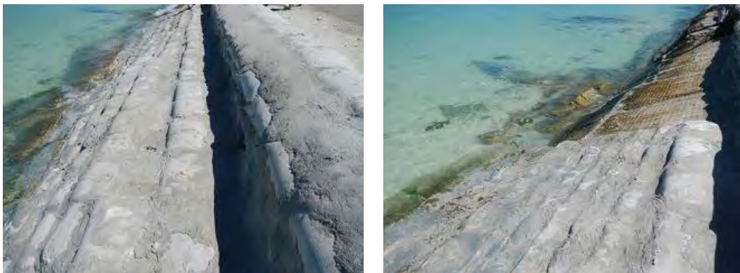
Repair of slopes
