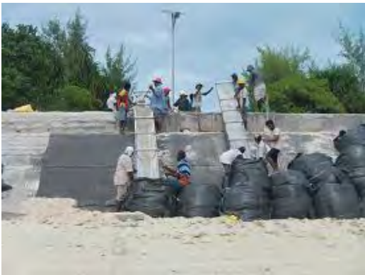
Installation of sandbags
