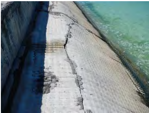
Peeling after application of mortar due to poor workmanship
