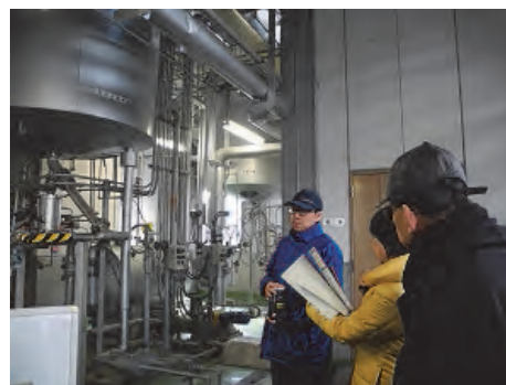
Photo 2.29 Training in Japan (Kyoto Municipal Waste Edible Oil Fuel Production Facility)
