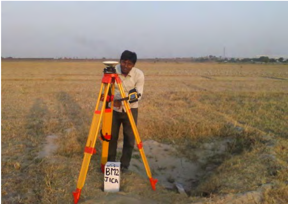
1. Photo no.1 shows DGPS Establishing a TBM.
