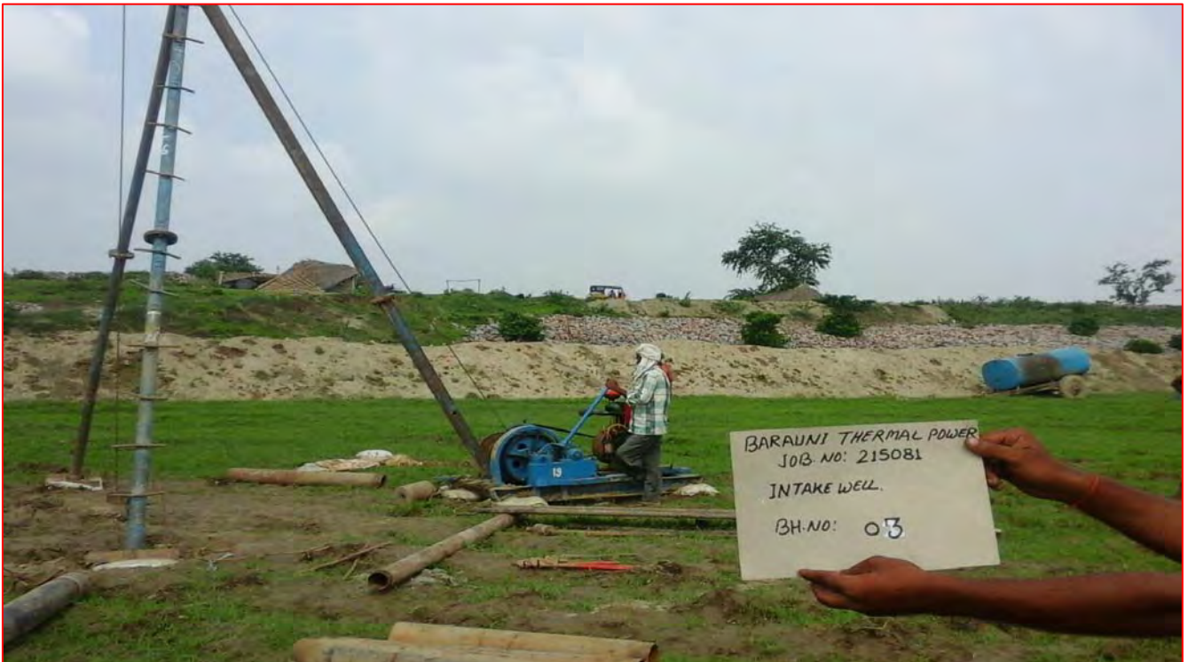
Photo: 2 Borehole No. BH-3
