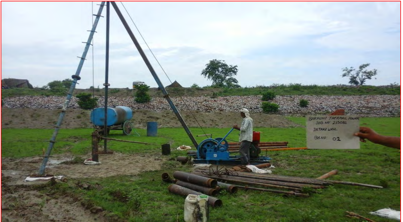
Photo: 1 Borehole No. BH-2
