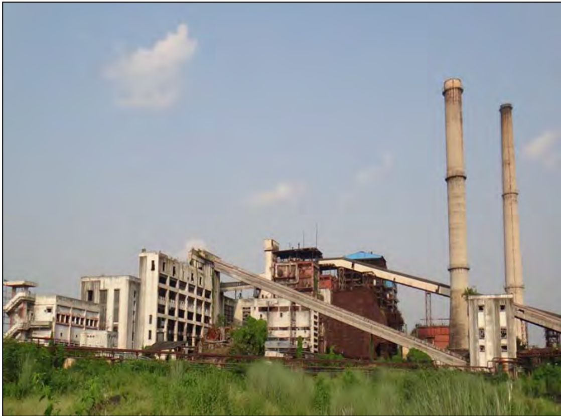
Figure 3.1-1 Distant View of BTPS (Unit No. 1 to 7)
