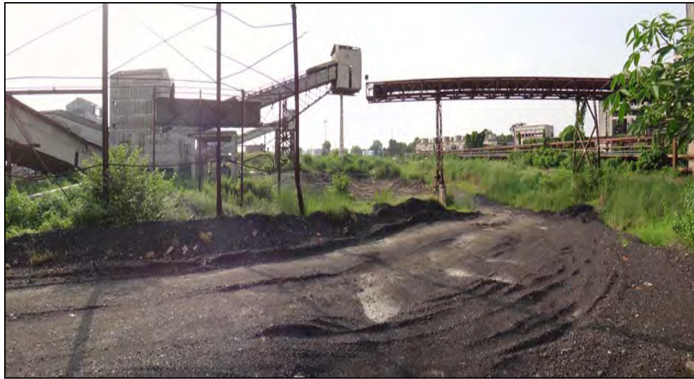
Figure 3.1-6 Condition of Coal Storage Yard
