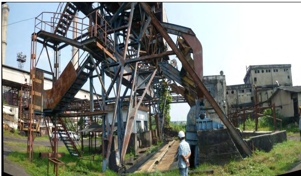
Figure 3.1-5 Wagon Tippers (Coal Unloading Equipment)
