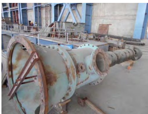
(Temporary storage of a pump on the turbine floor)
