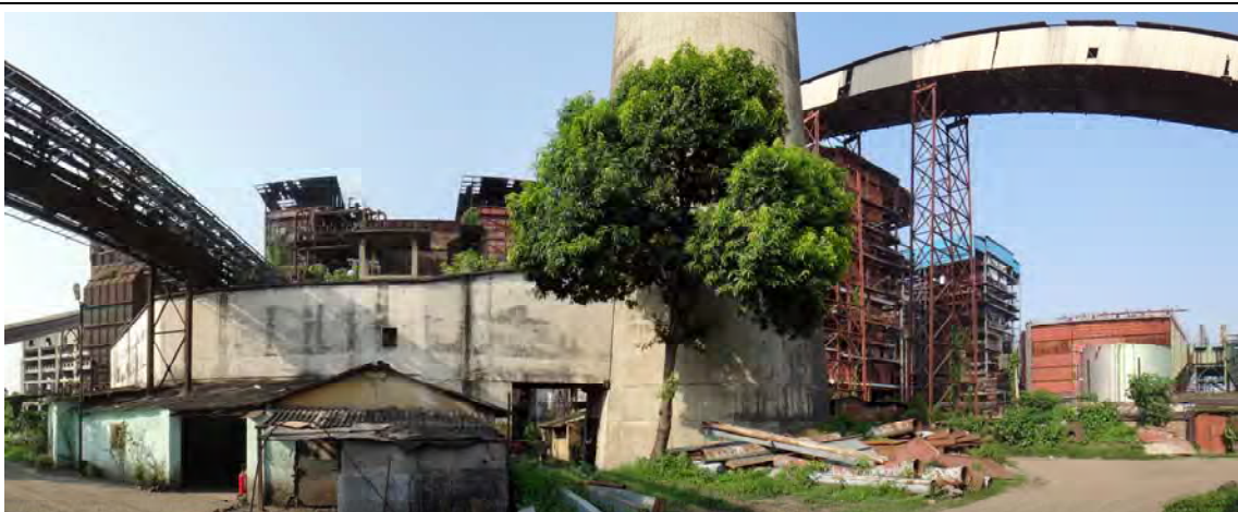
Survey of conditions at Units No. 1-3 (Units No. 1-3 turbine house)
