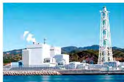
Reihoku I :SC Coal-fired TPS (1995-) Reihoku II :USC Coal-fired TPS (2003-)
