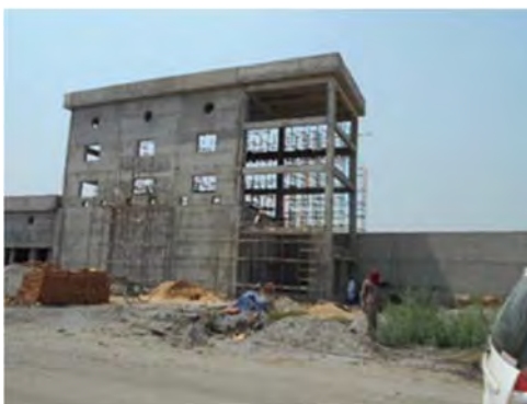
(Raw water storage tank)
