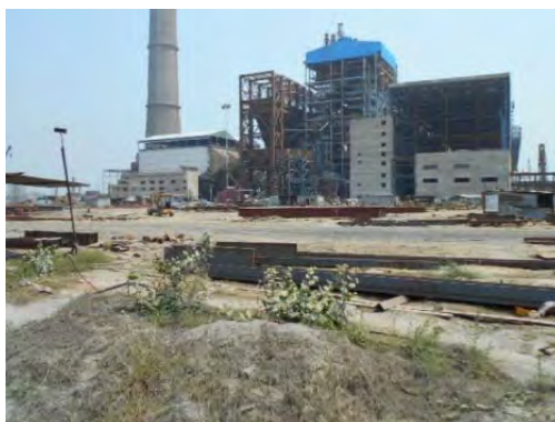
(Unit No. 10 construction area)
