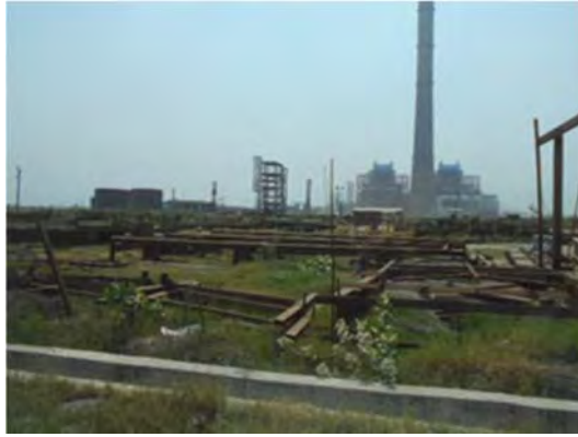
Equipment and materials yard near the stacker/re-claimer
